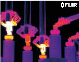
Thermal inspection of a high voltage installation.
